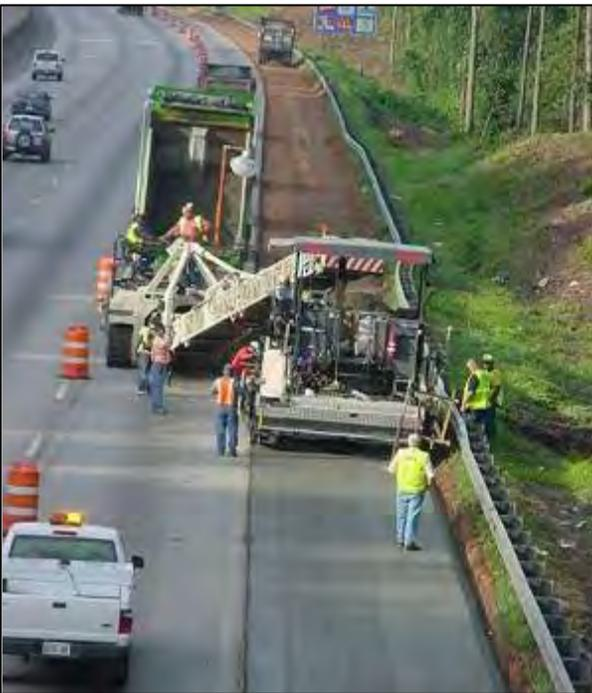
**Figure 9.** RCC construction.
