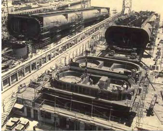
Figure 11-4 BART Tunnel, San Francisco
