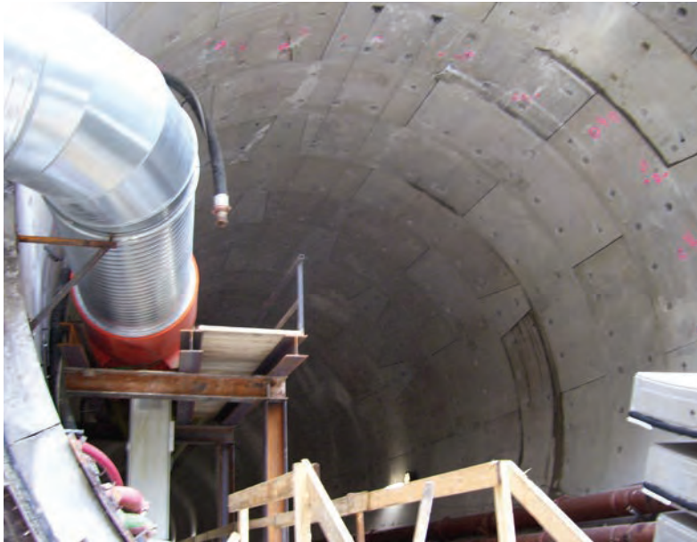
Figure 10-2 Precast Segmental Lining
