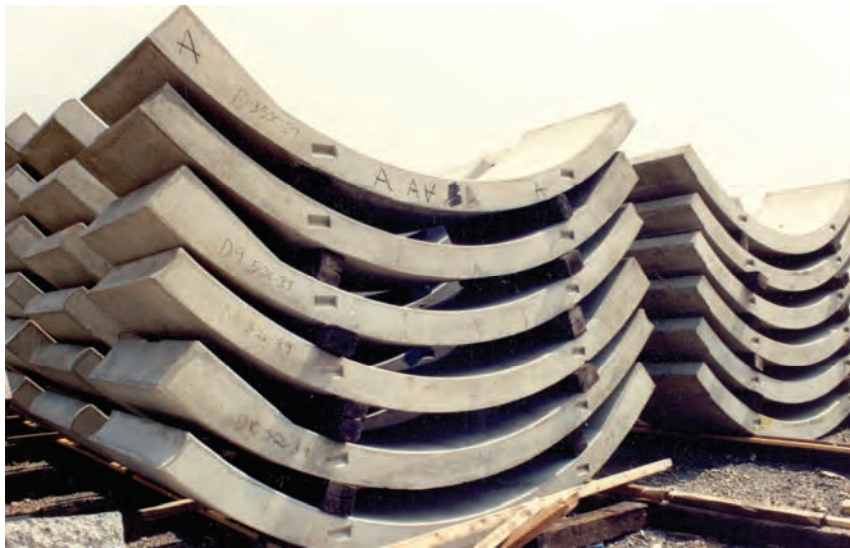
Figure 10-9 Stacked Precast Segments for Two-Pass Lining
