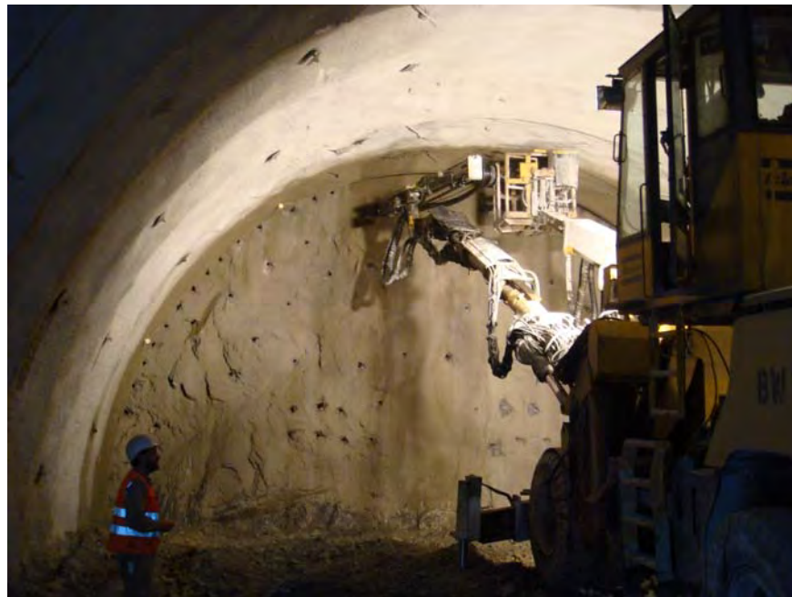
Figure 9-10 Face Drilling for Drill-and-Blast SEM Excavation (Andrea Tunnel, Austria)
