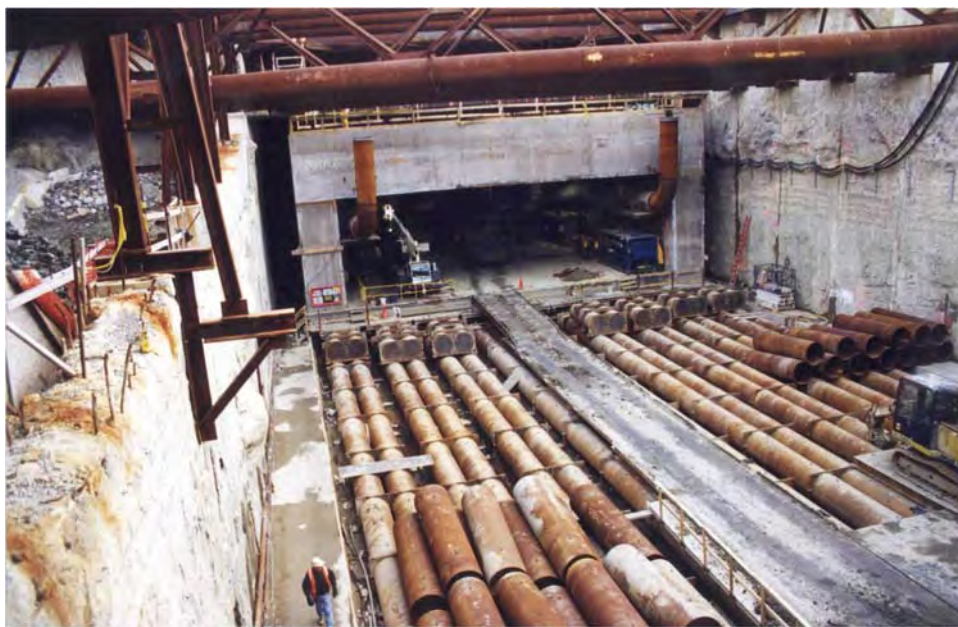
Figure 12-9 Progressive Installation of Packer Sections and Connecting Diaphragm Plates
