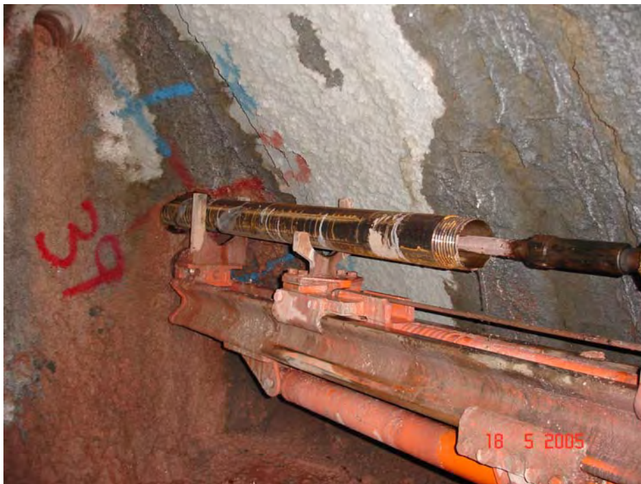
Figure 9-16 Steel Pipe Installation for Pipe Arch Canopy (Fort Canning Tunnel, Singapore)
