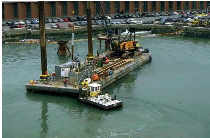
Figure 11-9 Fort Point Channel Tunnel, Boston
