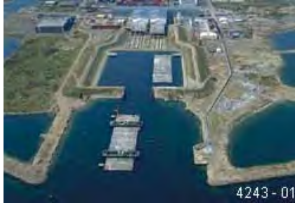
Figure 11-10 Fabrication Facility and Transfer Basin, Øresund Tunnel, Denmark
