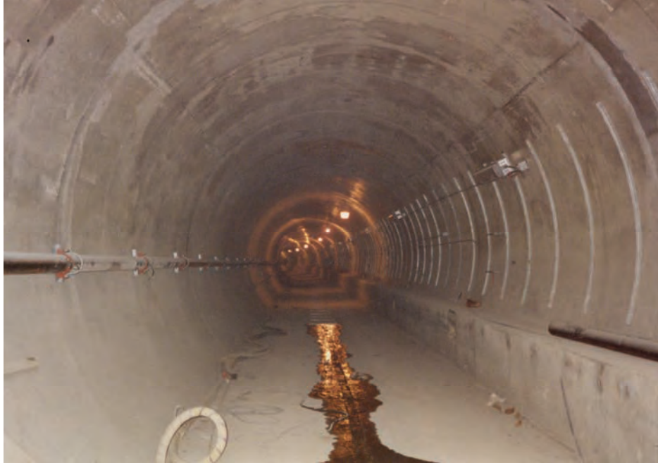
Figure 10-6 Cast-In-Place Concrete Lining, Washington DC
