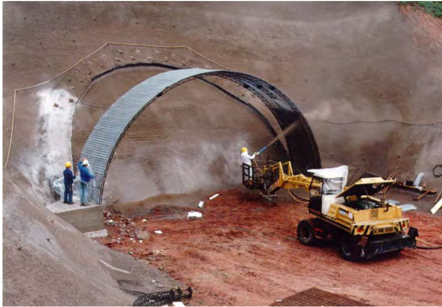
Figure 9-19 Shotcrete Canopy Construction after Completion of Portal Collar and Pre-support (Schürzeberg Tunnel, Germany)
