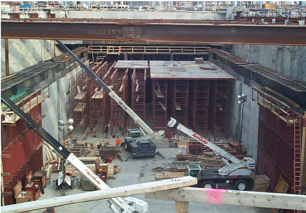
Figure 12-4 Tunnel Structure Construction Operation
