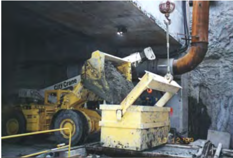
Figure 12-6 Scoop Tram Loading Excavated Material into Skip Bucket for Removal
