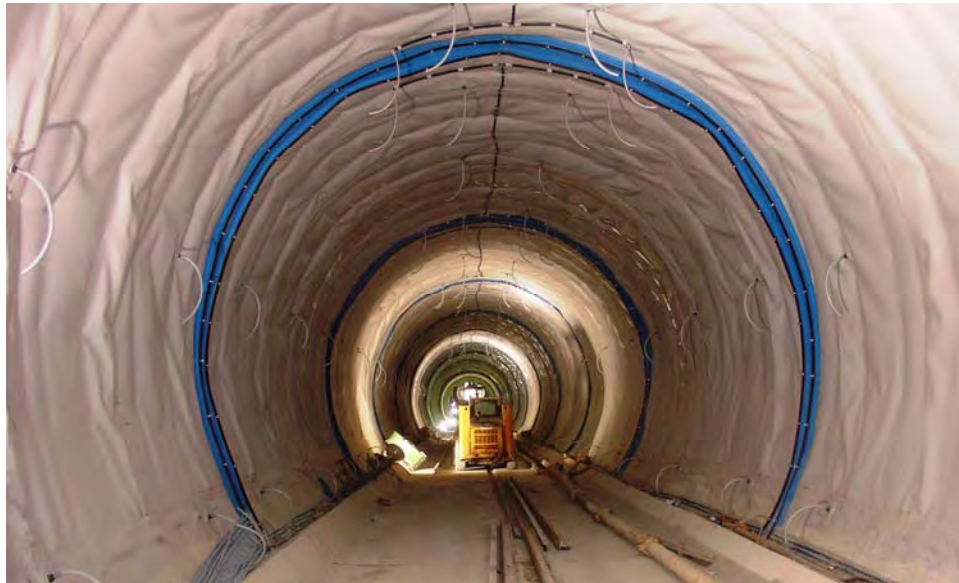
Figure 9-5 Waterproofing System and Compartmentalization (Automated People Mover System at Dulles International Airport, Virginia)
