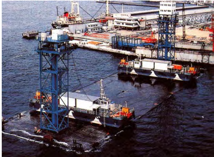
Figure 11-13 Osaka Port Sakishima Tunnel Element Transported to Site with Two Pontoon Lay Barges
