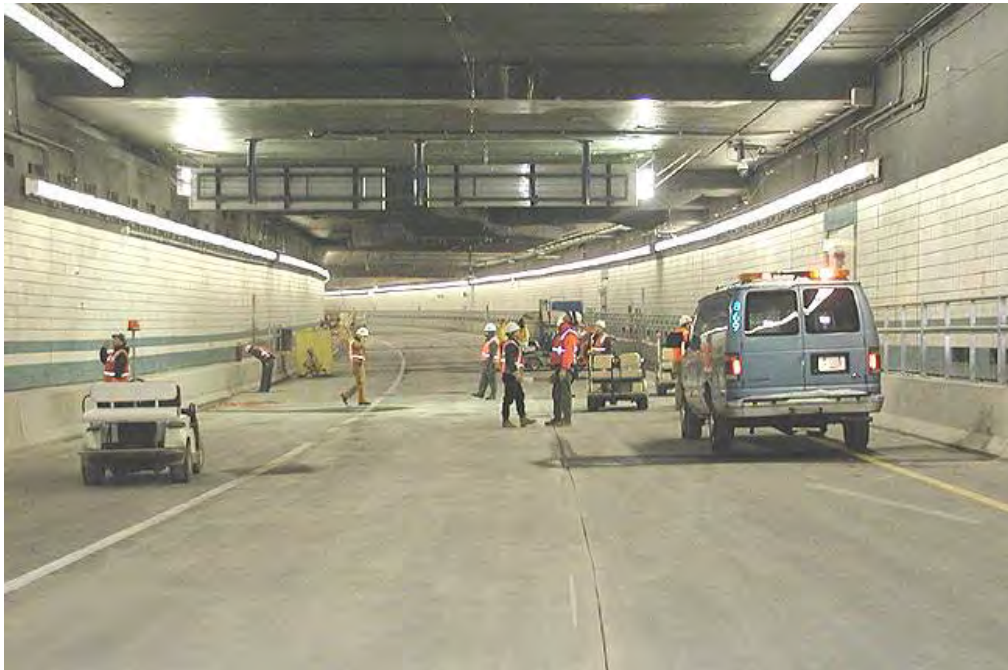
Figure 12-1 Completed I-90 Tunnels
