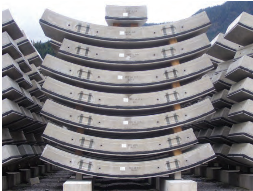
Figure 10-8 Stacked Precast Segments for One-Pass Lining
