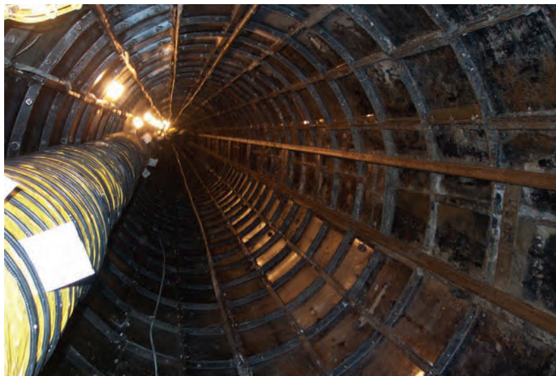
Figure 10-3 Baltimore Metro Steel Plate Lining
