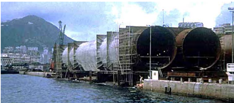
Figure 11-12 Hong Kong Cross Harbour Tunnel is Nearly Ready for Side Launching.
