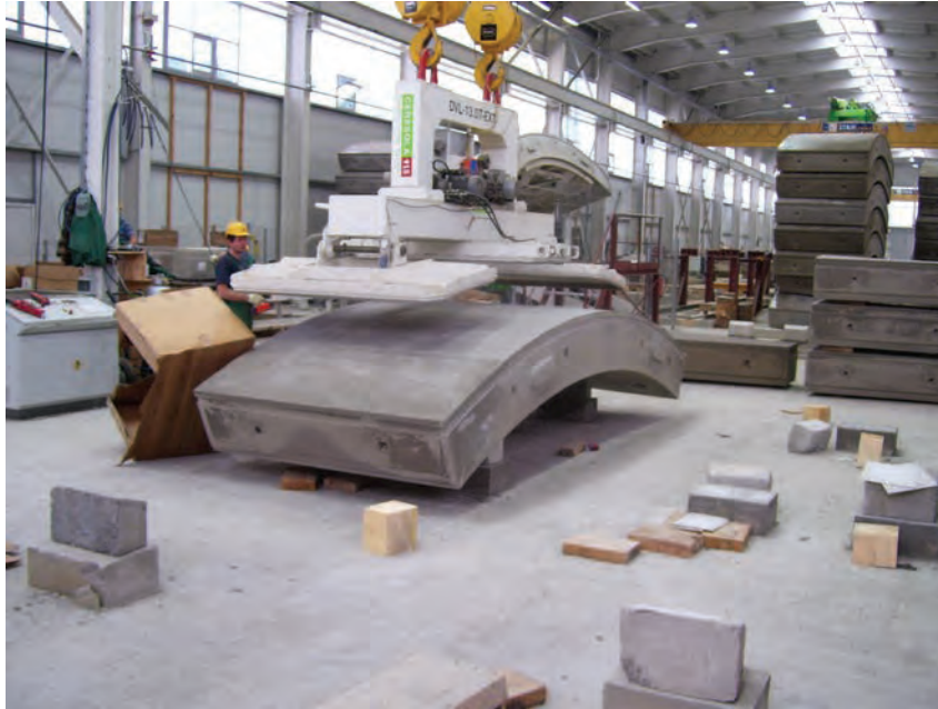
Figure 10-7 Precast Segments for One-Pass Lining, Forms Stripped
