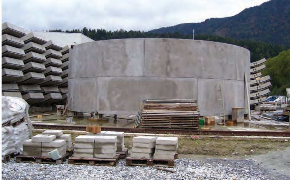
Figure 10-13 Mock-up of Precast Segment Rings
