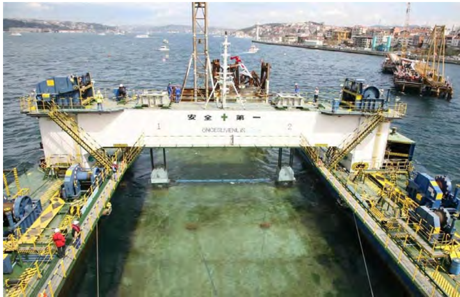
Figure 11-15 A Tunnel Element is Being Placed.
