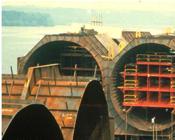
Figure 11-6 Fort McHenry Tunnel, Baltimore
