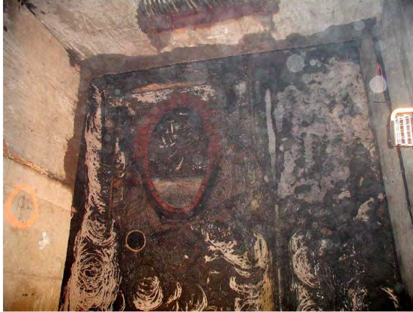
Figure 12-13 Frozen Face Seen from Shield at Front of Jacked Box Structure
