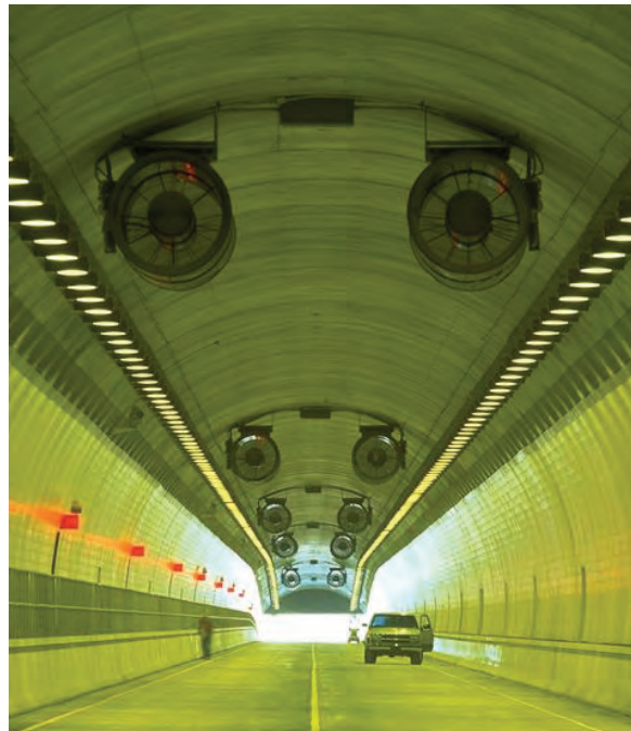
Figure 10-1 Cumberland Gap Tunnel
